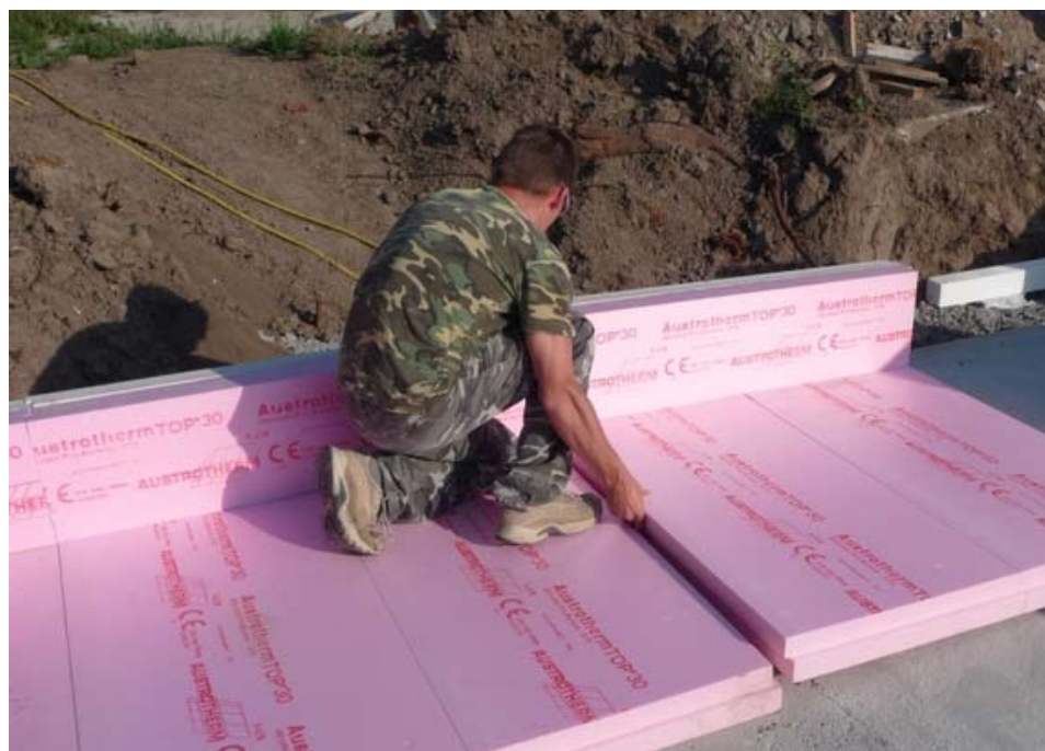
Austrotherm XPS a lemezlap alatt
